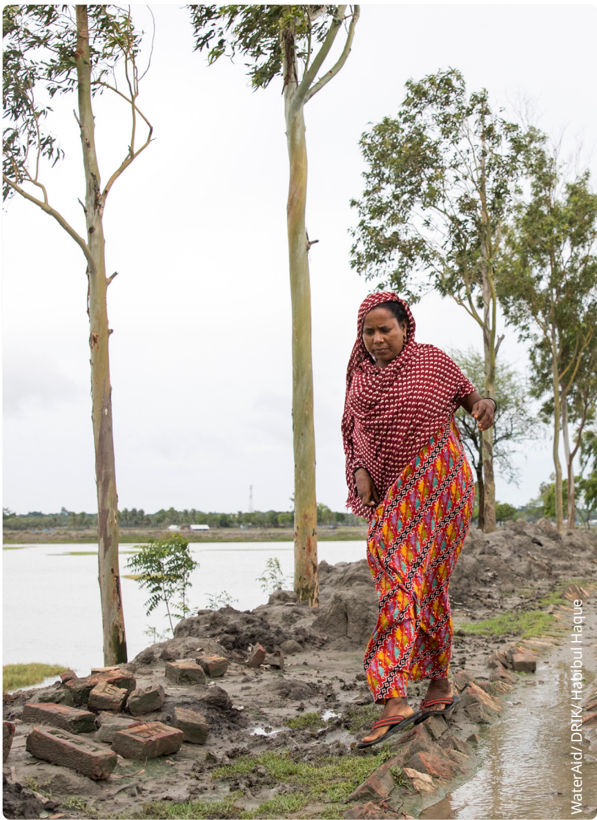
● Parul Begum, 35, walking through the damaged road near her house. Ward 9, Khulna, Bangladesh. September 2018.
